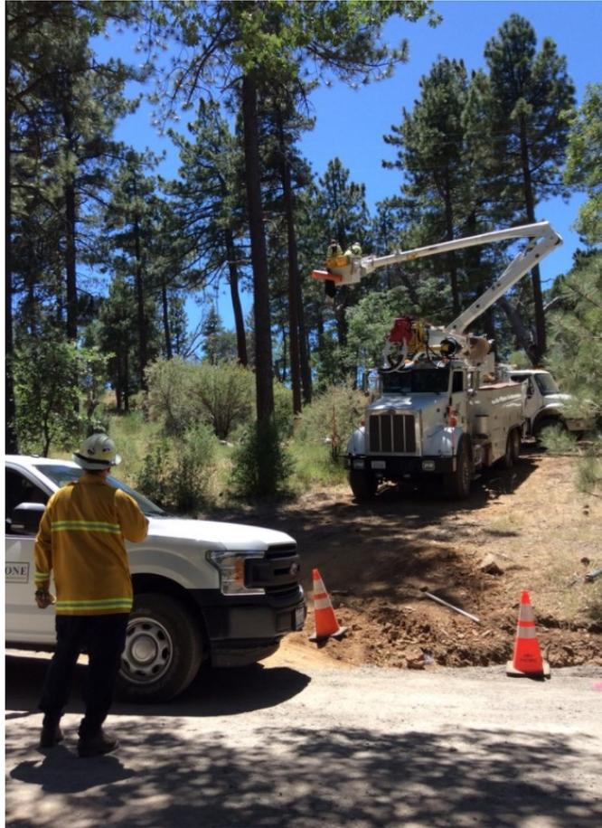
**Photo 5:** A Designated Fire Patrol was observed monitoring conductor work with de-energized lines at P260436 (C 440 Phase II) in accordance with the CFPPP Fire Prevention Matrix for the activity on USFS land with a PAL D (MM FF-1). A Project WEAP sticker was observed on the Fire Patrol's hard hat in accordance with MM BIO-2.
