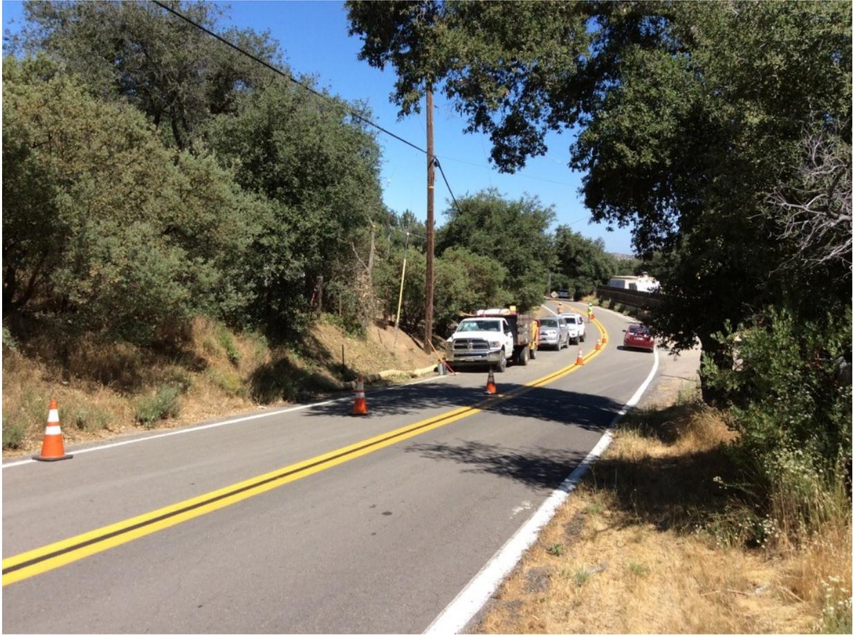
**Photo 6:** Cones, signage, and flagpersons were used to direct one-way traffic around the work area for Vault 71 and P259843 and P259844 (C 440) in accordance with the Traffic Control Plan (APM TRANS-05) and APM TRANS-02.
